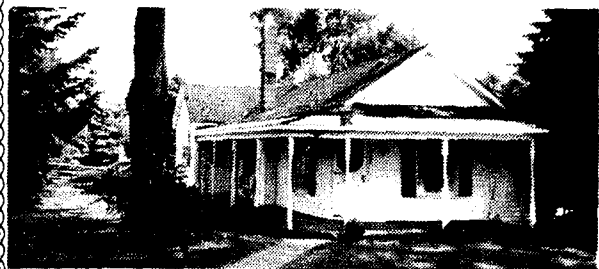
CL-470 FANTASTIC STARTER HOME or rental property. Across from the Village Park in Central Lake. Easy access to Intermediate Lake, downtown shopping. Cozy & comfortable. 24 hr. notice to show. $38,900.
