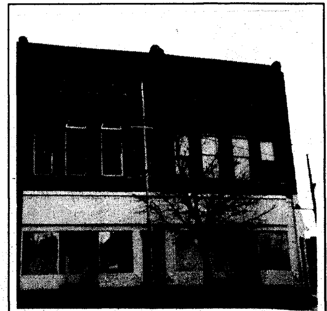
EMPTY BUILDINGS like these have contributed to a decline in local property values. East Jordan may soon have a Downtown Development Authority to take action in reversing the trend.
