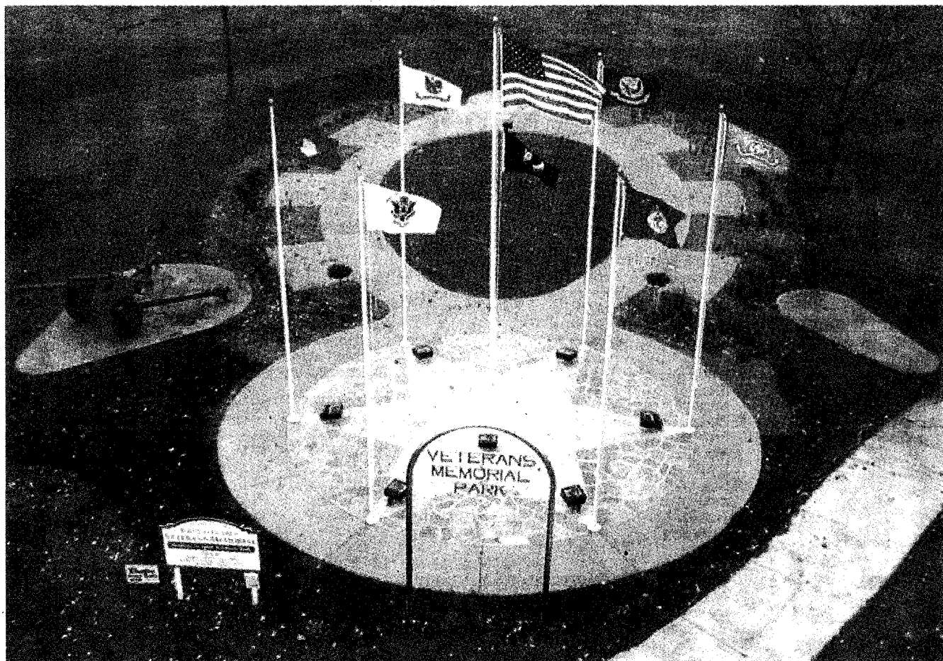
Work nears completion on the new Veterans Memorial in Veterans Park. With the installation of the flagpoles, the annual Veterans Day observance took place Nov. 11 at 11 a.m. The stonework will be completed in the spring. The WW II gun is completely restored and in place and the Civil War canon will be restored next.
