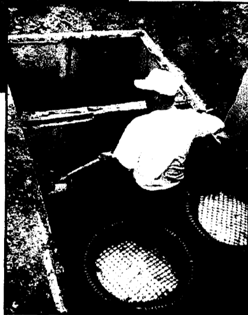
NSFC staff helps install an alternative onsite system in Benzie County, Michigan
