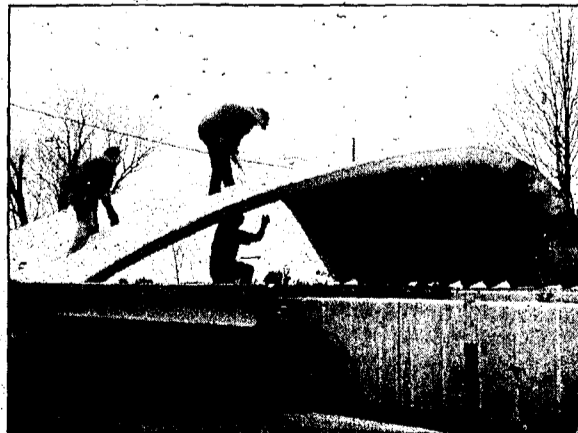
After Boyne City commissioners unanimously voted in the spring to remove the bandshell in Veterans Park, city crews had it down a few days later. The decision by the commission came after a long controversy over the bandshell which was built in the 1950s. "In the last five years, we've given it the very best and all efforts to bring the bandshell up to date have not succeeded," Mayor Eleanor Stackus said at the time of the vote.
