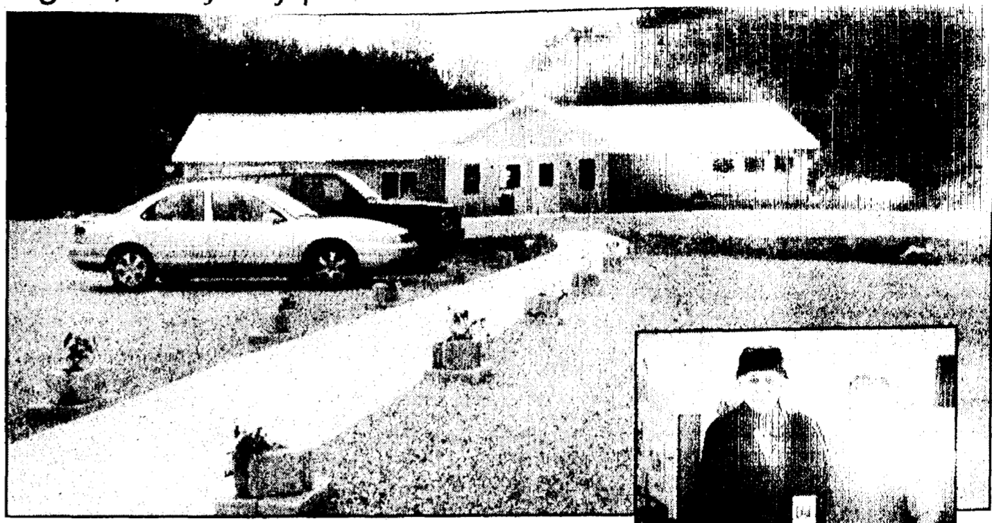
The new parking lot and entrance at Raven Hill was made possible by the generosity of donors, including $25,000 from Warren Loranger, right.
