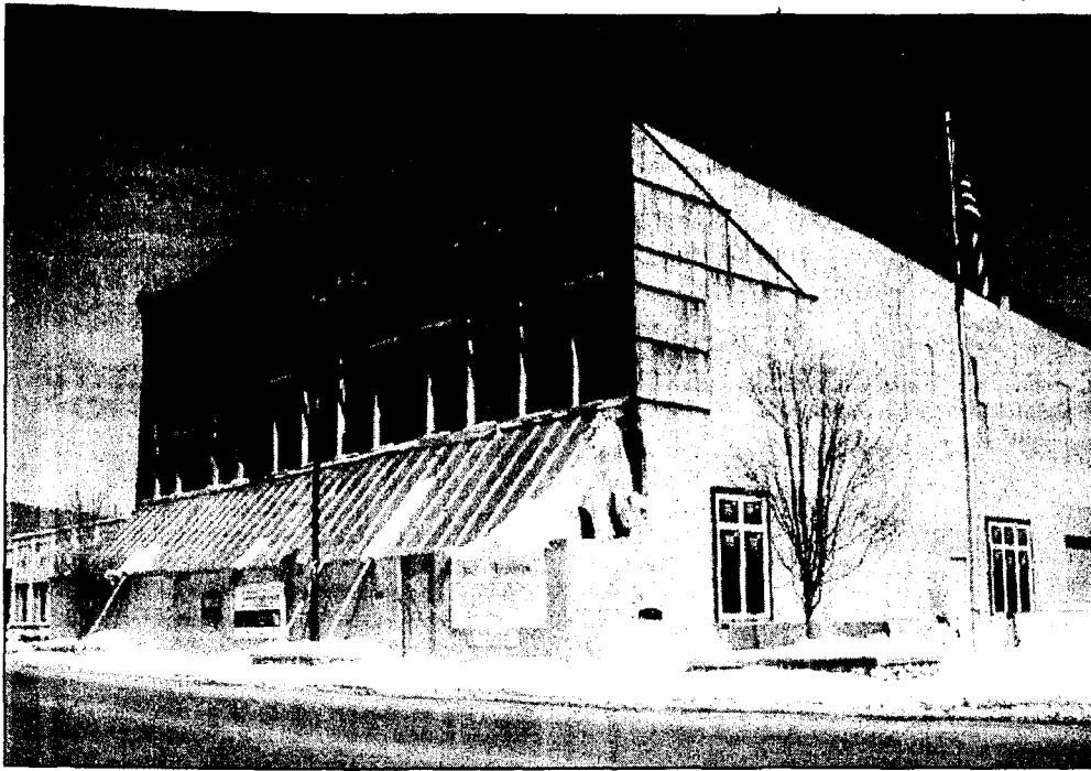
The face of the former Votruba and Porter Lumber buildings has undergone significant changes over the course of the last few months of construction under the watchful eye of developers Floyd and Todd Wright. The facade, above, has been partially obscured for several months as crews have worked inside; at top right, the original bricks on the south and east walls have had to be completely removed, leaving a blank slate. Brickwork is expected to begin within the month.
