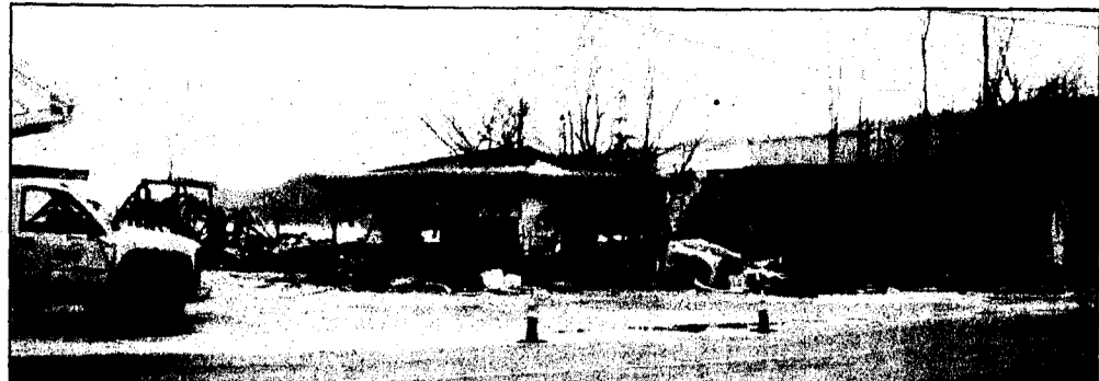
Last week's blaze left only a shell of what once was the Walloon Lake Marina. The fire melted cable and phone wires, leaving the village with no service until the next day.
