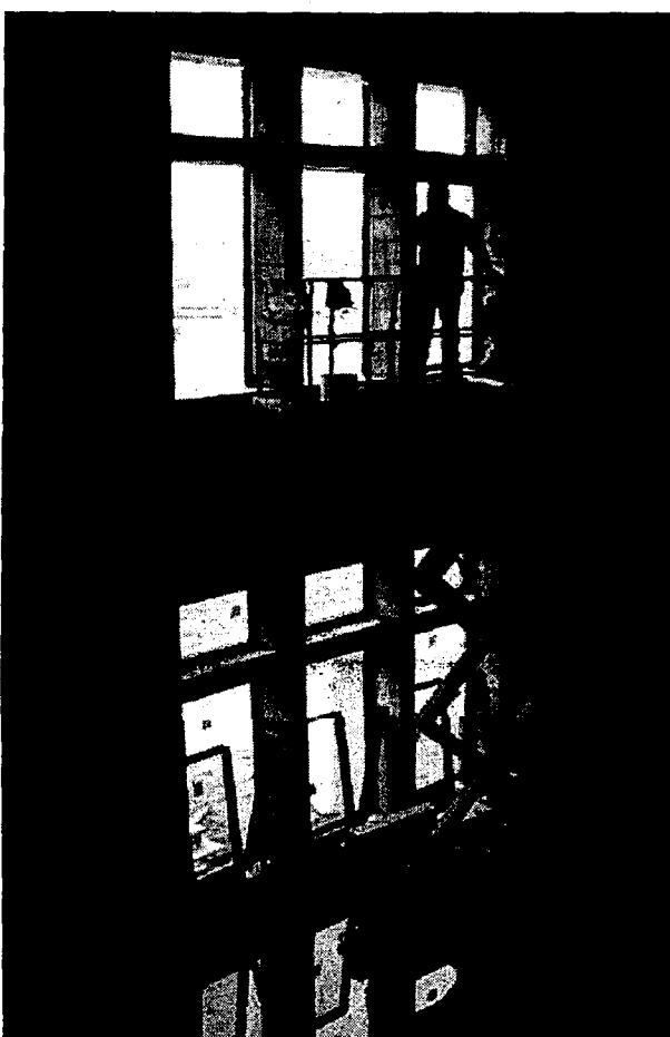
Work on the new Boyne City High School, to open for the 2002-03 school year, made great strides, rising from the landscape after extensive site preparation.
