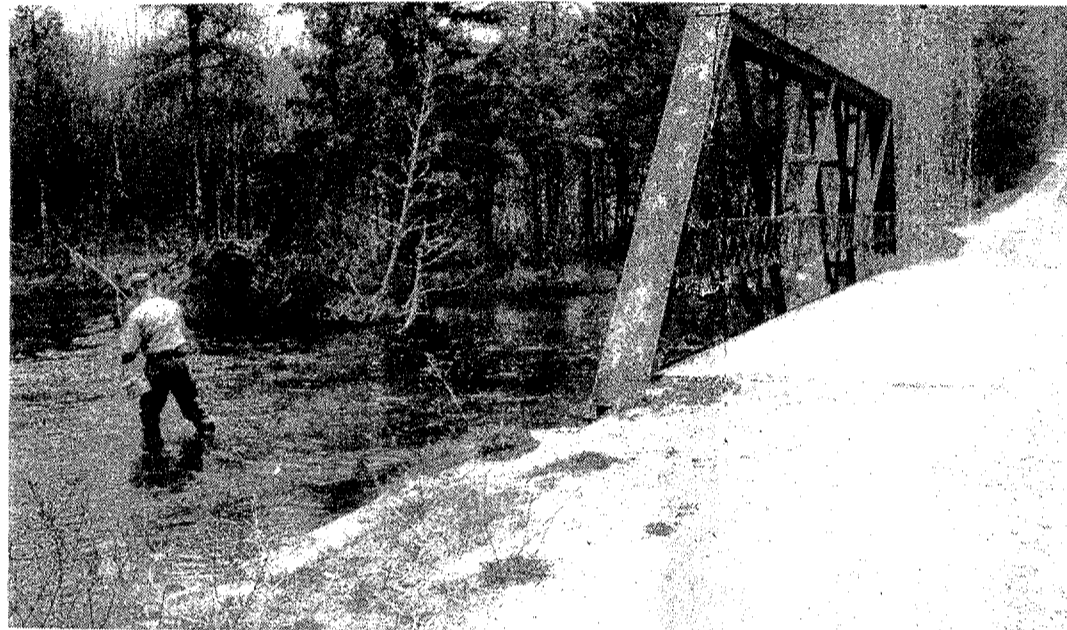
ORIGINALLY built around 1900 for logging, Pinney Bridge, at M-66, is a fly fisherman's paradise.
