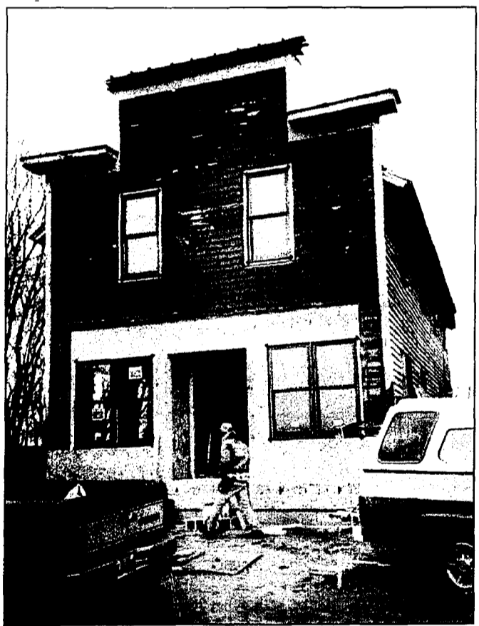
A volunteer work crew recently installed new energy-efficient windows and doors at the Jordan River Watershed Center.
