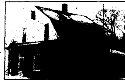
Much of this house on Third Street in East Jordan was destroyed in a fire last week.
