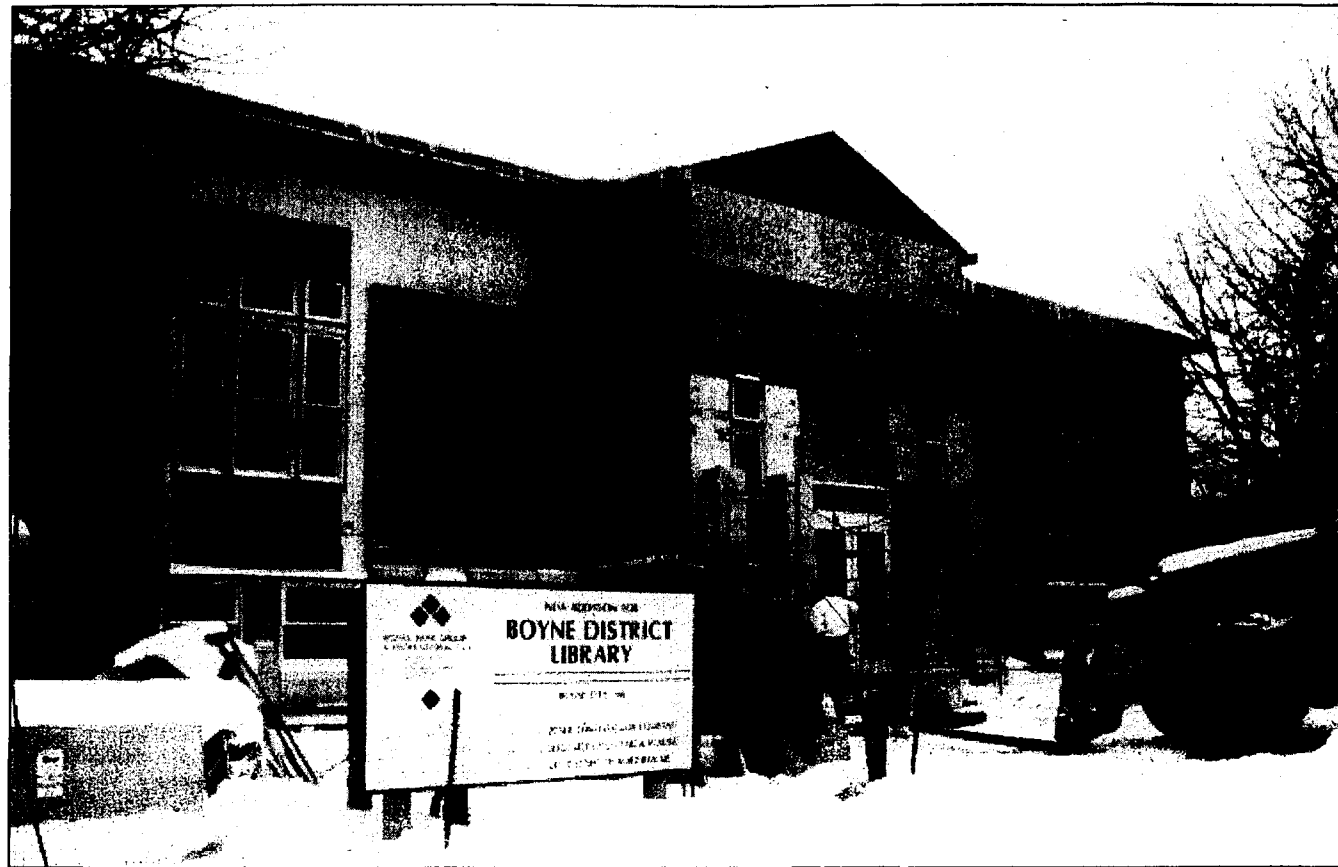
The new main entrance for the Boyne District Library faces Park Street, and is rapidly taking shape as work moves ahead.
