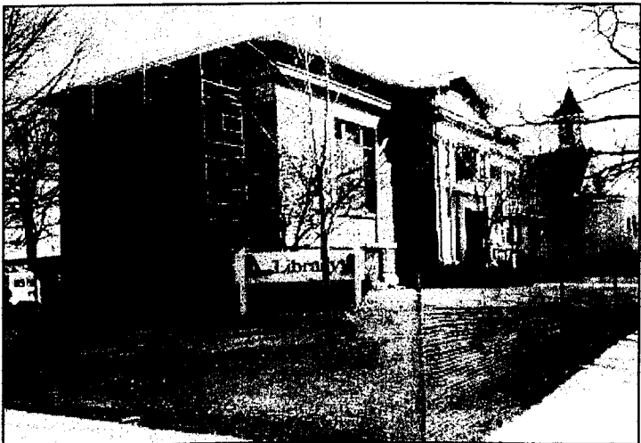
In March, work began on an extensive renovation and addition to the Boyne District Library.
