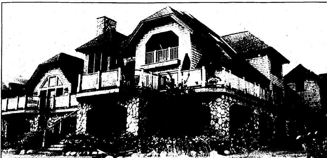
Pat and Gerry Carroll's waterfront home was designed by architect Douglas Wright, and built by Floyd and Todd Wright.
