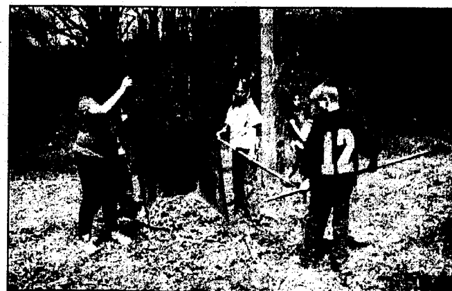
East Jordan sixth graders spent some time last week constructing a ropes course at the middle school. Pictured, from left, are Amanda Klitson, Nichole Crain, Bridget Knight, and Andrew Wiser.
