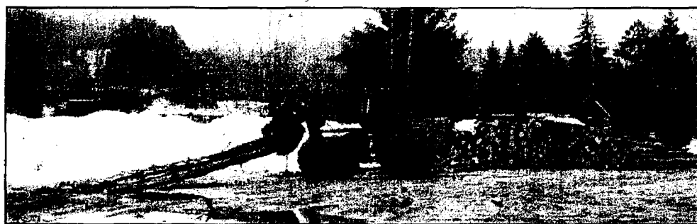
Tree removal is the first phase of the site development, with electrical preparatory work scheduled to begin soon.
