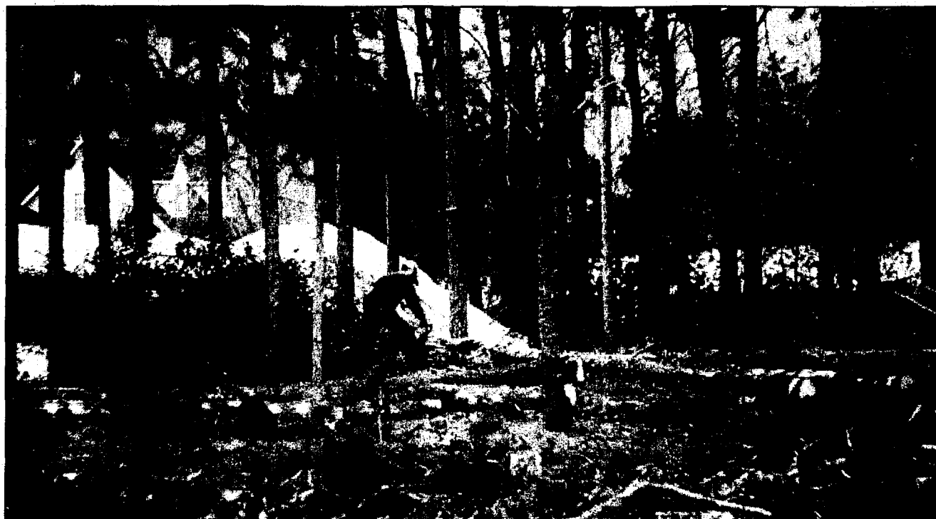
A worker prepares logs for removal from the site of the new high school in Boyne City.
