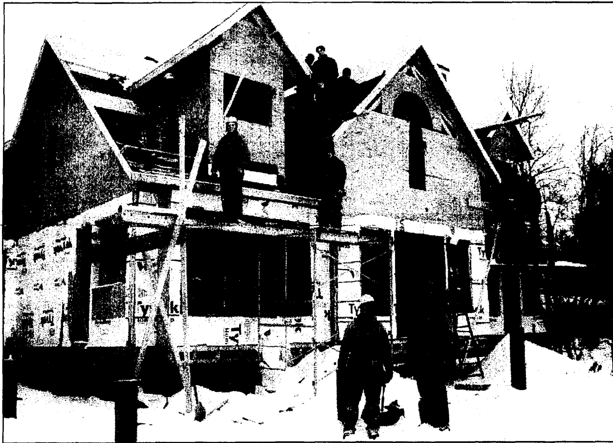
Boyne City High School teacher Tom Neidhamer and local contractor Nord Schroeder, foreground, are supervising 16 students on this year's Building Trades home, located on Deer Lake.
