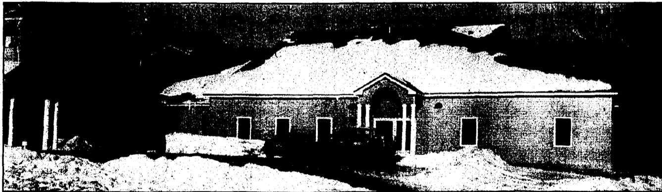
Concord Academy Boyne's new addition will house six classrooms, a staff lounge, and a performance room. They hope to be moved into the space within the next month.
