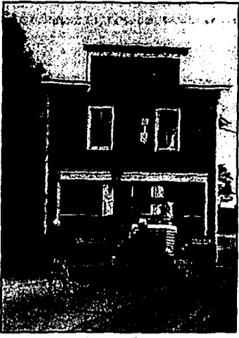
Slowly and carefully, movers ease the old Trading Post building onto the highway.
