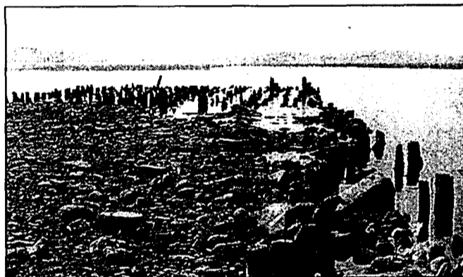
Lower water levels reveal old pilings and a part of Boyne City's history. The pilings are in front of the One Water Street Restaurant.
