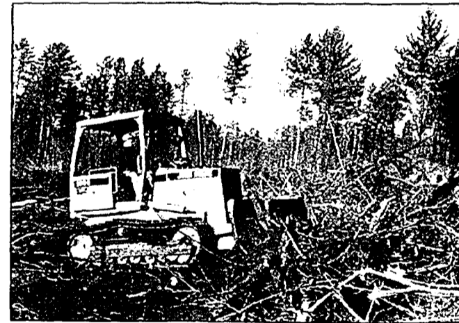
Timber was cut and cleared from Boyne City's Rotary Park to make room for new softball, baseball and soccer fields. Work will continue in the spring.
