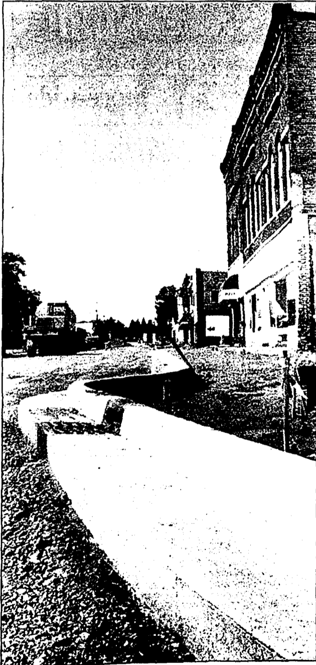
East Jordan underwent its first streetscape renovation in nearly a century, bringing a new Main Street, sidewalks and curbing, from Mill to Garfield streets, to the city's downtown. The $2 million construction project, which began in the spring and was completed in the fall, included new storm sewers, watermains and sanitary sewers, and a facelift for Esterly and Spring streets. The finished-off "Up North" look features fieldstone planters, turn-of-the-century style lighting, and specialty landscaping.
