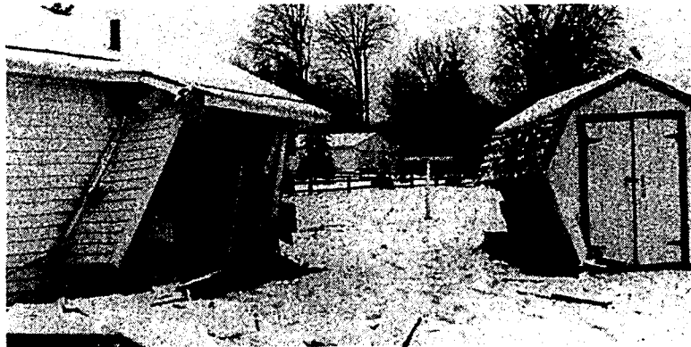
Damage galore was left behind after a vehicle smashed into the side of a house on Lewis Street early Monday morning. Ann Ketchman was sleeping inside at the time of the accident, but she was not injured, only startled.
