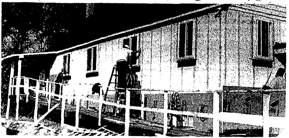
Work on the church included installing new windows, siding and insulation.
