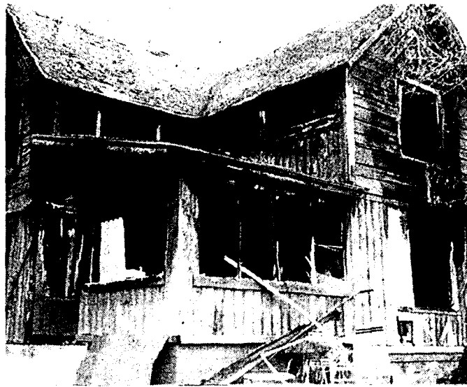
A fire destroyed this home near the elementary school in East Jordan last week.
