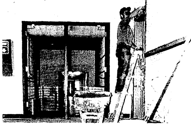
Petrie Construction carpenter Chris Derenzy builds a door-frame at East Jordan Elementary School. Part of the facility is undergoing renovations this summer.
