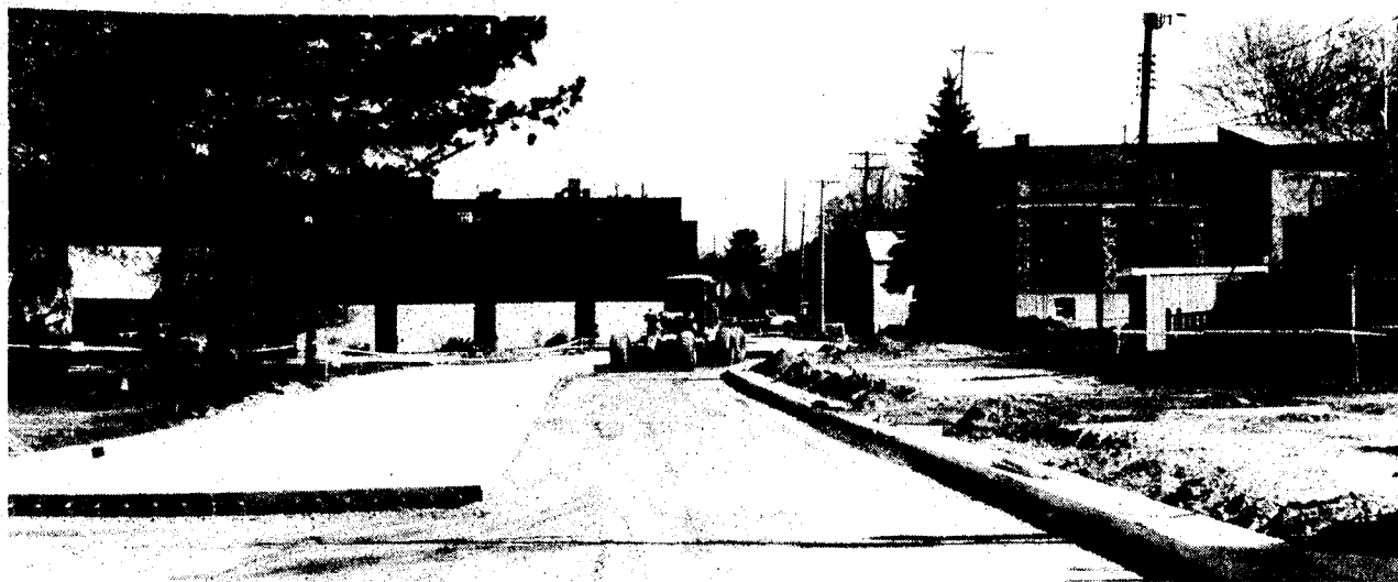
Concrete was poured last week and after 30 days of curing, East Jordan's Spring Street will be open to traffic.
