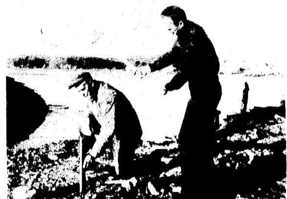
Richard Sligh pounds in a stake held by Bret Riley as the men stake out location of a new building at East Jordan Marina.
