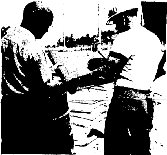
Frank Bretz, church construction superintendent, checks blueprints on the job with builder, Harry Watson.
