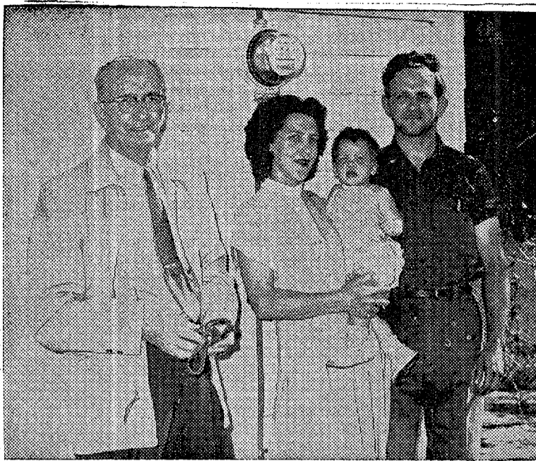
When the 10,000th meter was installed on the farm home of Ted Kucharek, Route 2, Gaylord, it made the Top O'Michigan Rural Electric Company, serving 12 northern Michigan counties, the largest rural electric organization in the United States north of Kentucky. On hand to congratulate the Kuchareks were Manager Harold S. Lees, left, Mrs. Lois Kucharek, their daughter Tonya, and Ted Kucharek.
