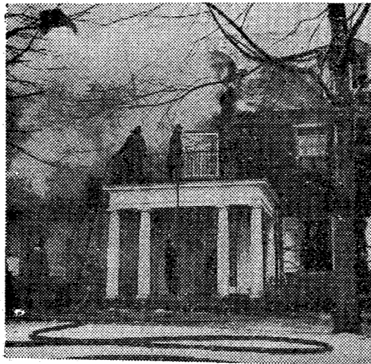
They did not get their chimney fixed when it began to spark ...
