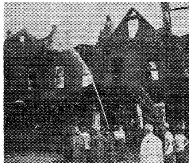
This homeowner put too many appliances on one electric outlet ...
