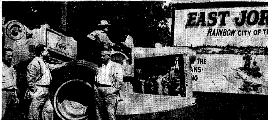
Historic moment: Giant earth moving equipment went to work at the site of East Jordan's new industrial plant, Aug. 16. Seeing a dream become a reality were from left: Albert Sinclair, president, East Jordan Industrial Development Corp.; Mayor Chris Taylor; and M. N. McDaniel, chairman, East Jordan Businessmen's Association.
