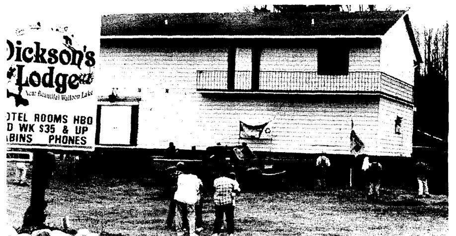
The newest additions to Dickson's Lodge will increase its room capacity by 34. Some of the rooms will be ready for occupancy by June.
