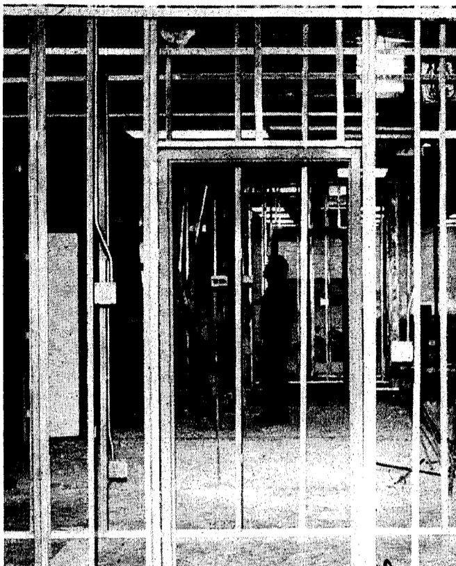
New classroom walls are taking shape at East Jordan Elementary School. The target date for completion of the project is mid August.
