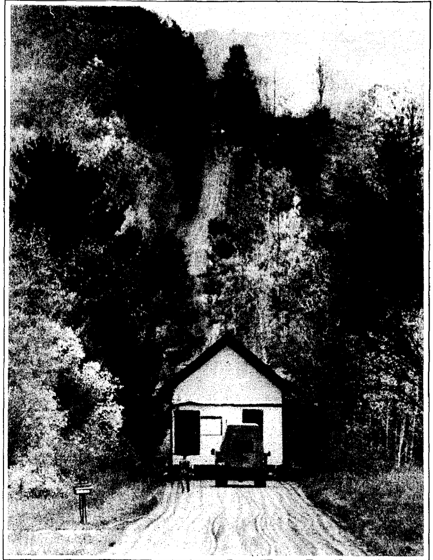
The old Wilson Township Hall found a new home at Raven Hill Discovery Center. The greatest challenge moving the hall in October was navigating the steep hill on Fuller Road.
