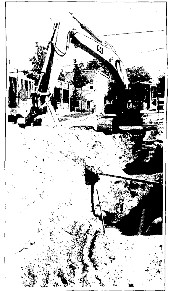
Projects got underway in downtown East Jordan as the Downtown Development Authority began implementing its long-range plan. The city will also be getting a new police department building in the coming year.
