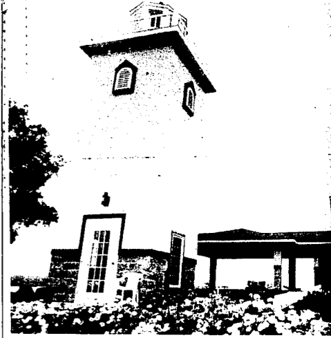
An addition was made to the Boyne City marina facility during the construction of the new marina facility/light tower.
