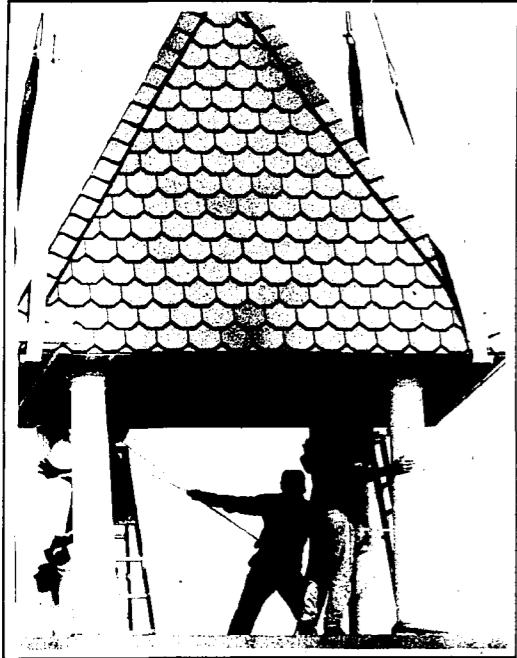
With the tower hanging in the air, workers carefully guided it into place on the new Tower Center in downtown Boyne City. The building has been renovated into four retail businesses and is home to Roast & Toast of Boyne and Kilwin's.
