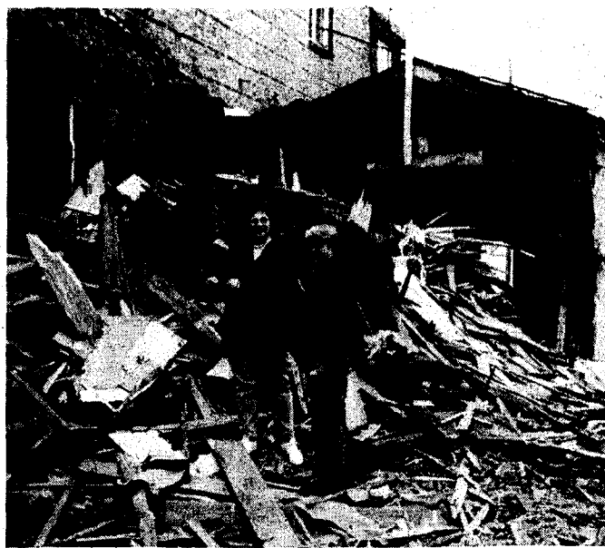
Jeannie Alward, left, and Cathy Cohen stand in the rubble of the old building that was demolished on the property where their new store will be in downtown East Jordan. The back of the store will house the Jordan River Fly Shop, run by Cathy's brother-in-law, Bob Cohen.
