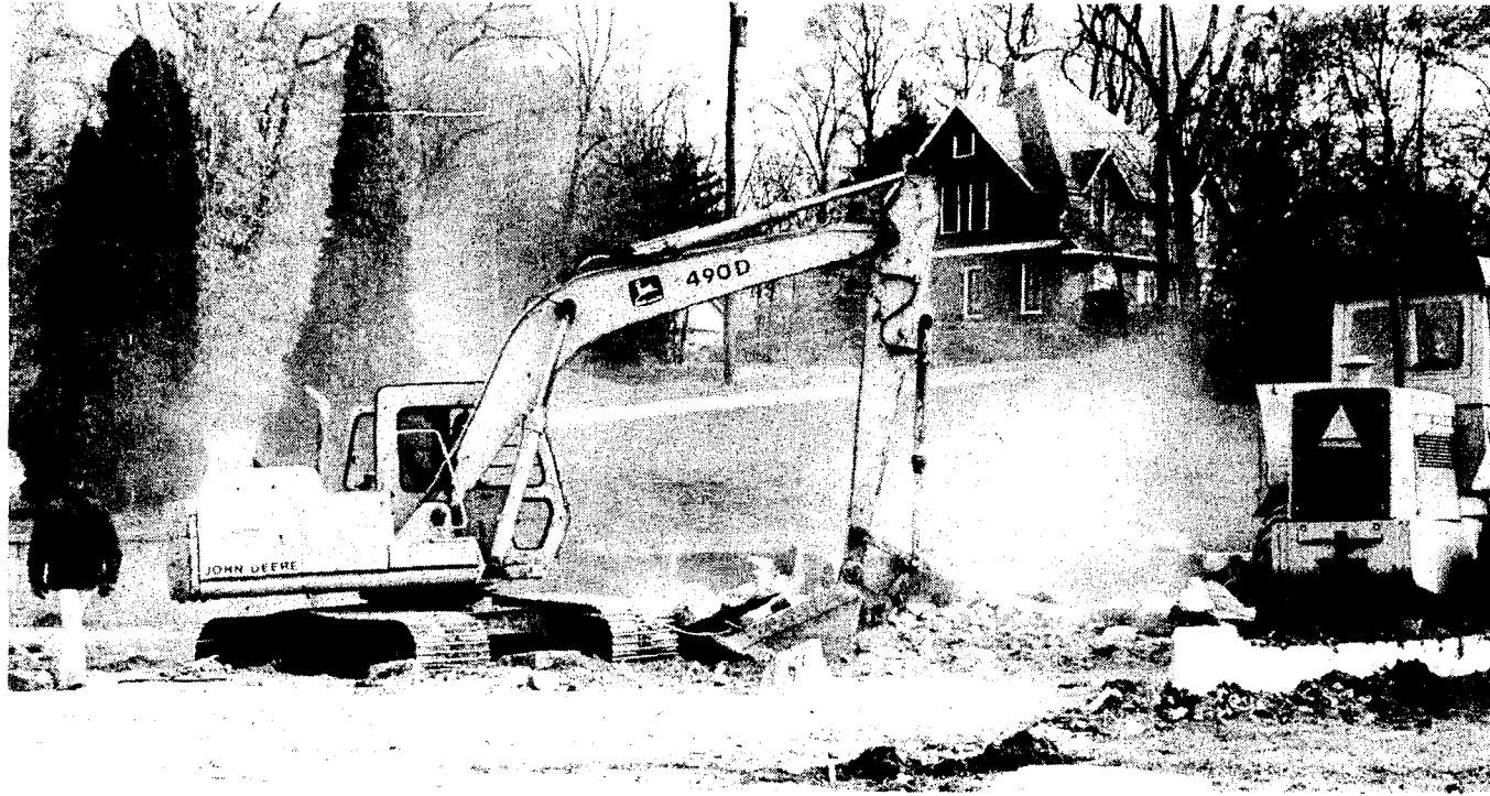
Spike's gas station and garage on the corner of Main and Garfield streets was torn down last week. This is where East Jordan's new police station will be built in the spring. Workers from Bartlett Excavating of East Jordan made the dust fly as they broke and shoveled pieces of concrete off the site.
