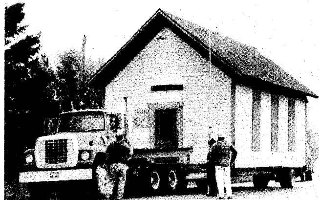
Top O' Michigan assisted with the move by raising power lines along the route.
