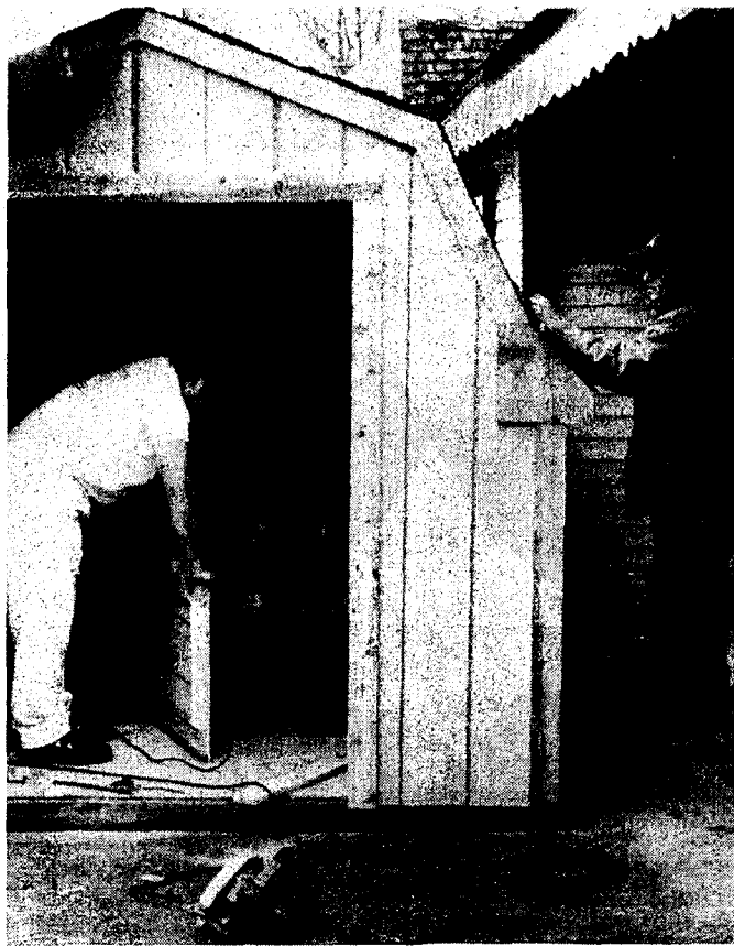
Boyne Area Head Start has a new storage shed, built by prisoners from the Charlevoix County jail. Materials for the shed were purchased by the school.
