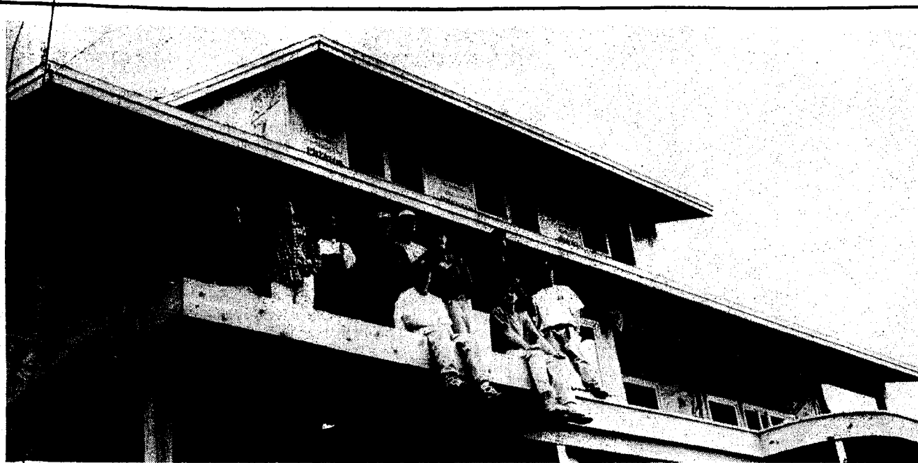
One of the features of Mike and Mary Long's new home is a deck which overlooks the Boyne River. The Building Trades Class will host an open house May 28 from 4-9 p.m. The home is located at 810 State St.
