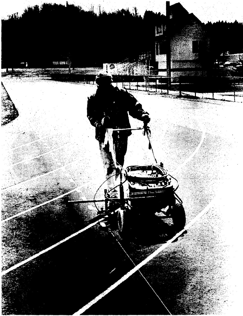
David Dinnocenzo, of Portland, Ore., was striping the track at the Boyne City Sports Complex last week. The temporary stripes will allow the track to be used this season, which begins Thursday. The track will receive its rubberized surface this summer.
