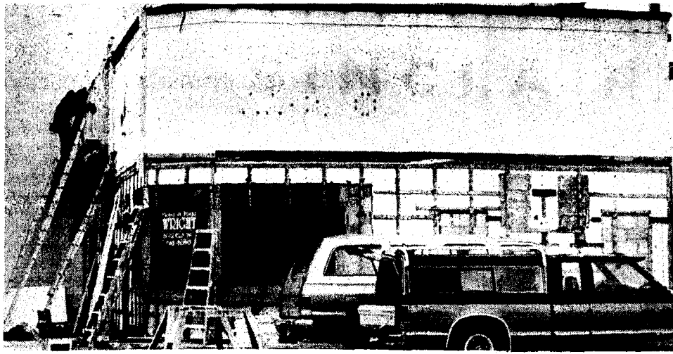
When the old facade was torn down, a sign from the past was revealed at the old Korthase-Lindsay building.
