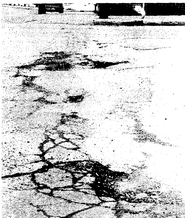
Potholes, like these at the corner of Main and Mill streets will be but a memory once the DDA's improvement project is complete.
