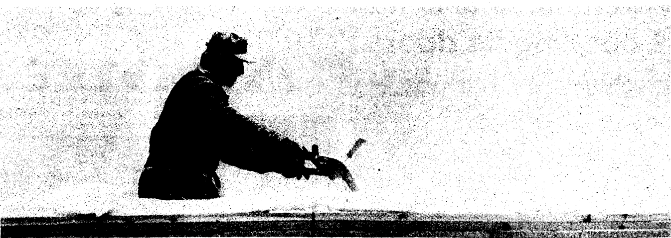
Bill Hawkins was creating his own blizzard last week, blowing snow off the new Boyne City Middle School gym roof. Hawkins Brothers Roofing is one of the subcontractors working on the gym.
