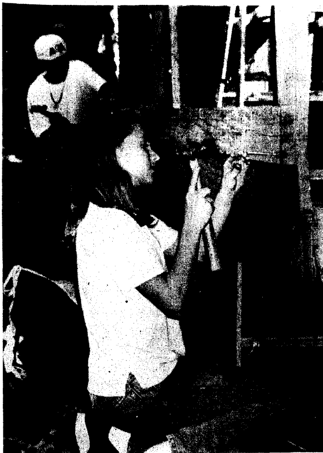
With hammer in hand, Jenny Barrow pounds a nail as The Wall begins to take shape.
