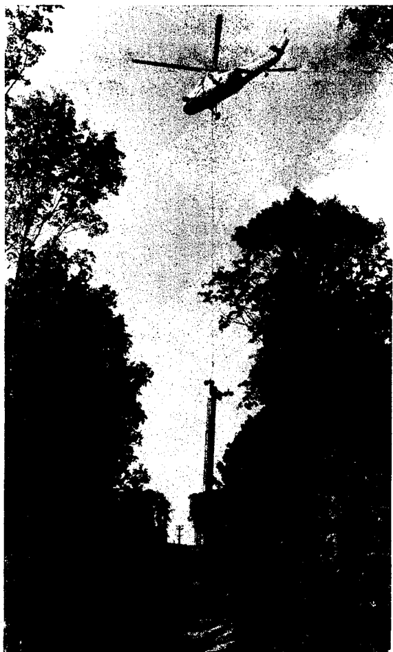
After its short flight, the helicopter moves the tower into position on Disciples Ridge.
