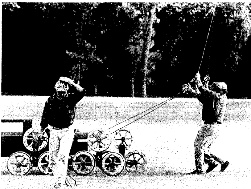
While the cable is connected to a tower.
