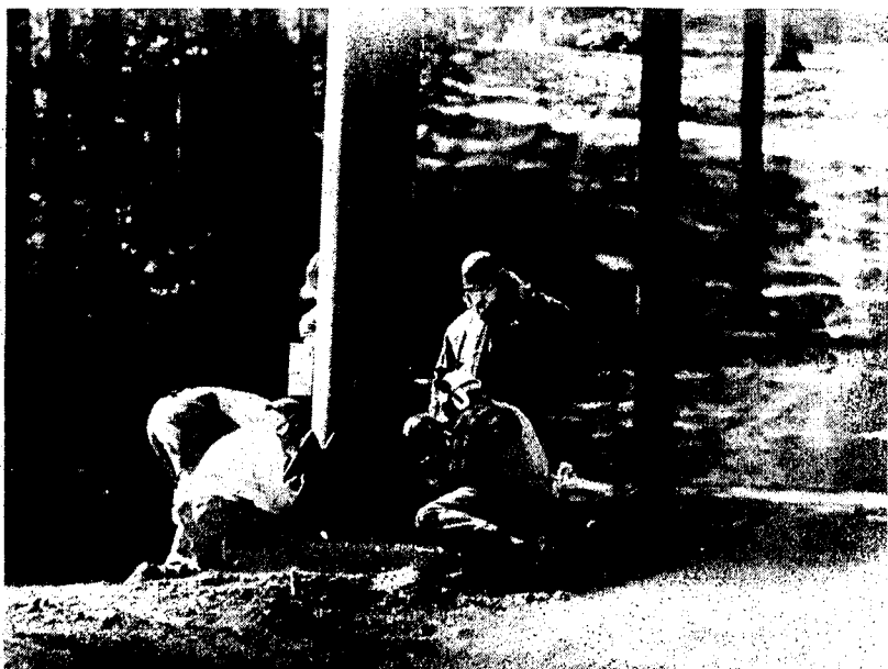
As dust flies around them, the crew works fast to bolt the tower.
