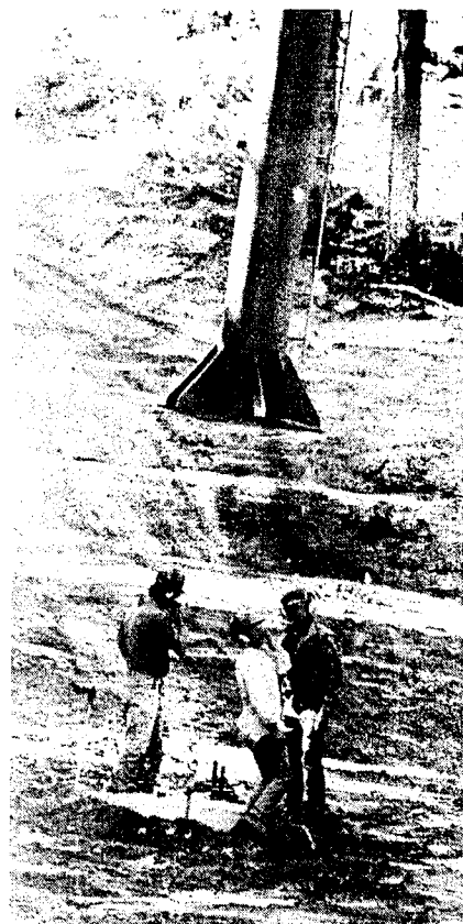
Like a big foot ready to step down, the tower comes within reach of the workers who will secure it to the concrete pad.
