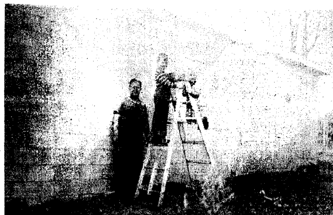
Allie stands by as Cecil and Phillip Chipman help build the new office and service building on State Street
