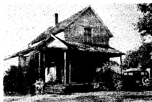
Starting out of this house on Vogel Street, the Chipman's built one of Boyne City's most successful plumbing and heating businesses
