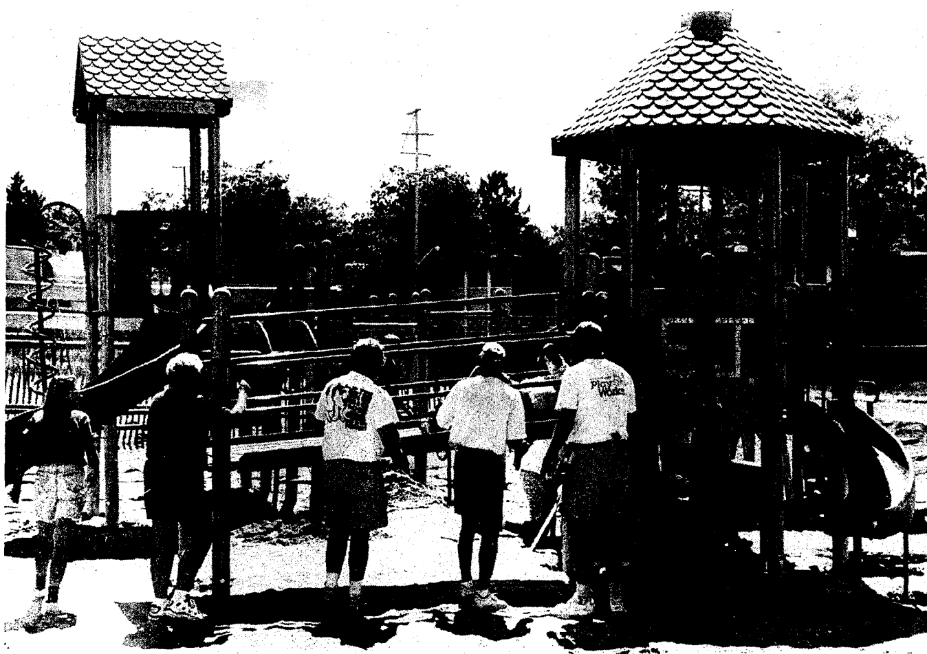
Volunteers spent the weekend erecting the new "Play Station" at the East Jordan Elementary School.
