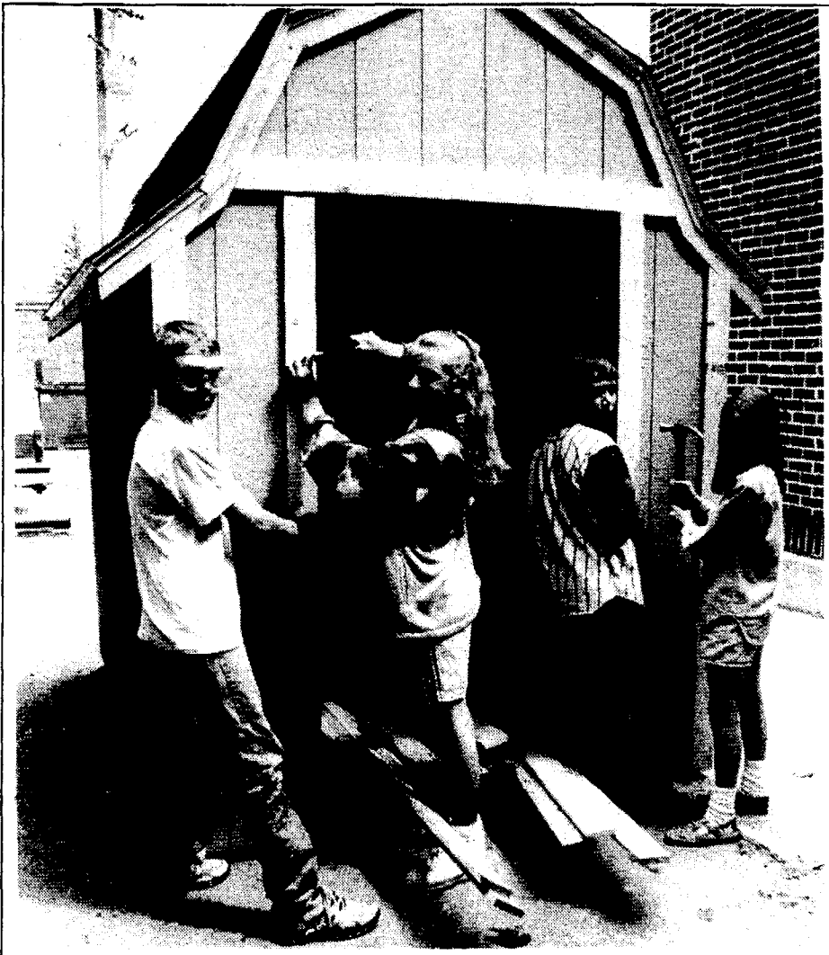
EAST JORDAN FIFTH-GRADERS learned a valuable assortment of skills while constructing this handsome shed. Working on the project are (from left): Mike Bartz, Stefanie Skop, Scott Pinney, and Destiny Bowman. The shed will be sold to the highest bidder and proceeds donated to Habitat for Humanity.
