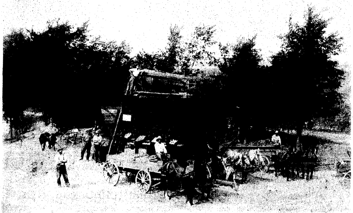
With all of the construction happening in Boyne City, we thought this picture of a gravel and stone separator back in the early times of the century was appropriate. This picture shows the machine in use with teams of horses and wagons getting filled up from the appropriate bin. Think how long the
