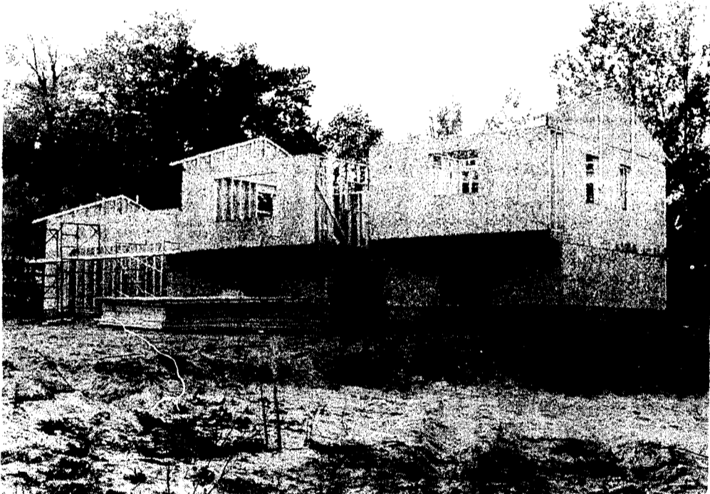
This home under construction by the Boyne City High School Building Trades program drew the ire of a local contractor who told board members the school should not allow a speculator to build a home for profit using student labor and not having to pay normal business expenses a regular contractor would have to absorb.
