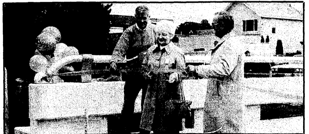
Cutting the ribbon to open the still uncompleted bridge was symbolic at best. The bridge work is expected to be completed in a few more days as the curb and gutter crews are preparing for paving of the new structure. The cost of the bridge is being paid 90 percent by the
